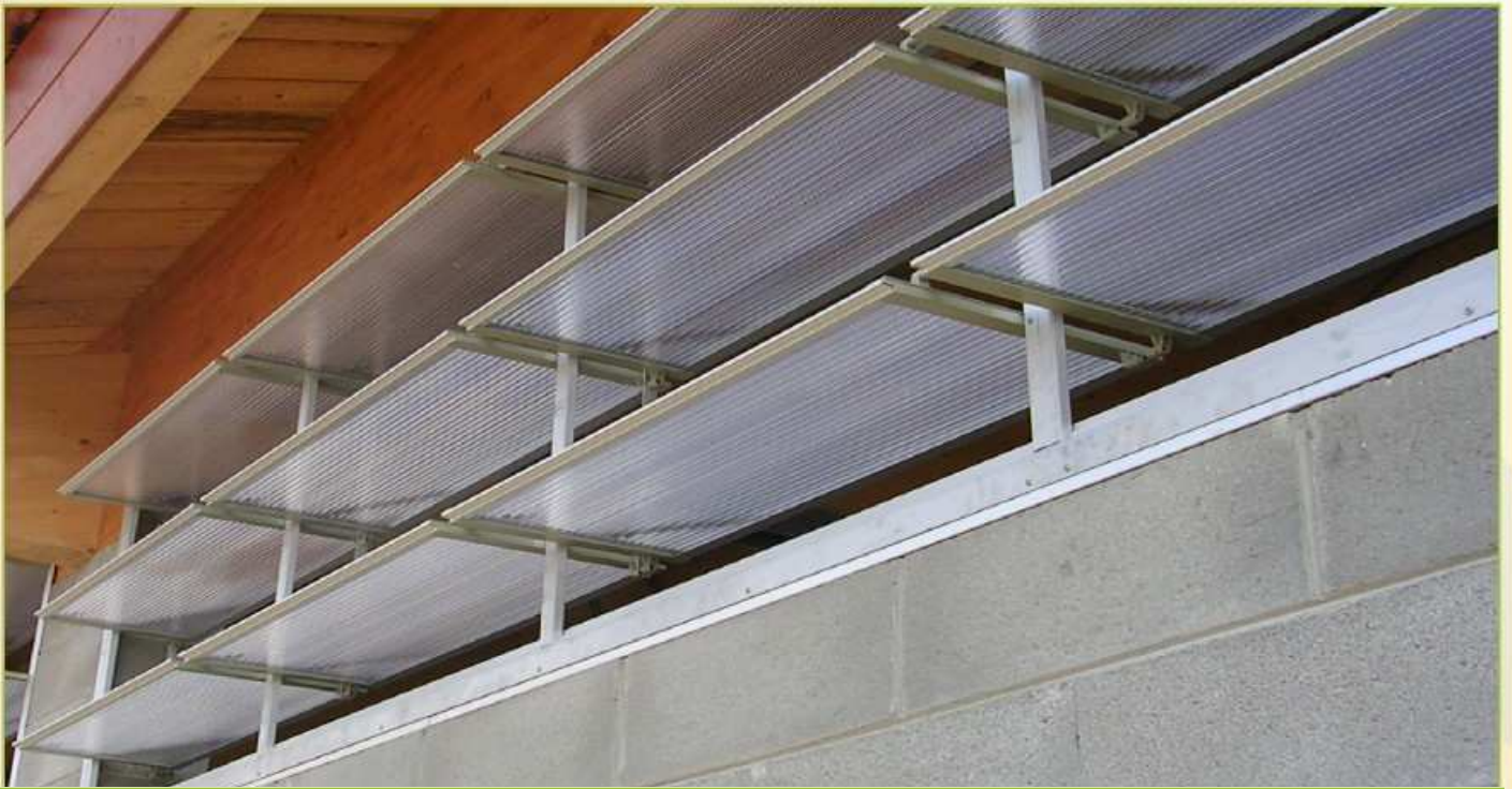
Parete trasparente apribile composto da pannelli modulari in polycarbonato Vertical transparent opening wall composed of modular polycarbonate panels
