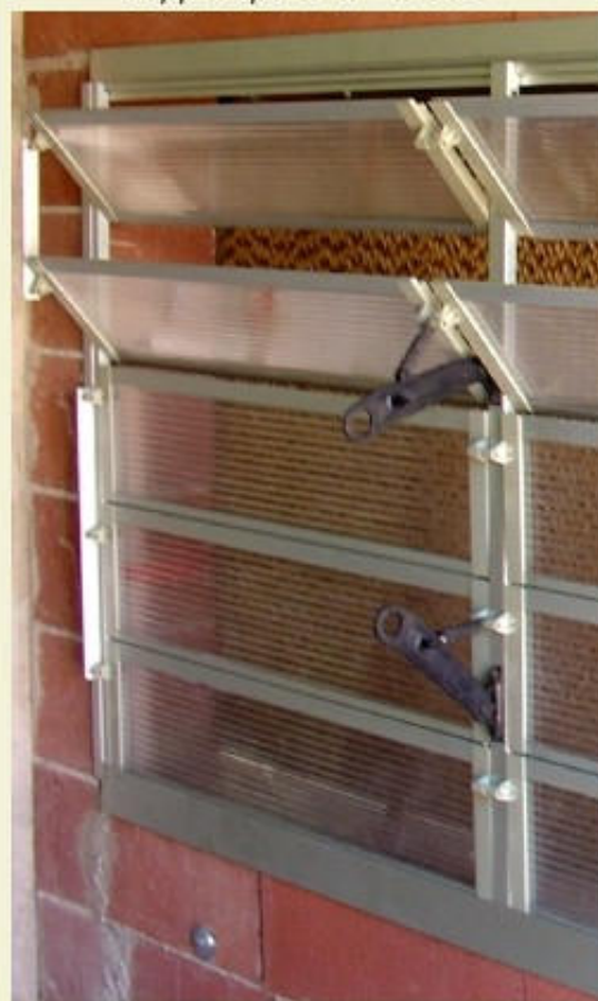
NW1B in front of cooling pad and double manual opening NW1B con pannello cooling e doppia apertura manuale
